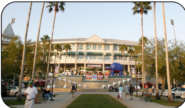
HAMMOND STADIUM - LEE COUNTY, FLORIDA
